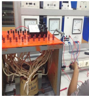
b) Finished transformer on tests with various meters
